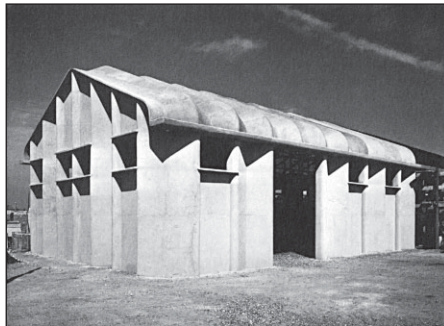
Fig. 3: The experimental warehouse in ferrocement, La Magliana, Rome, 1945
